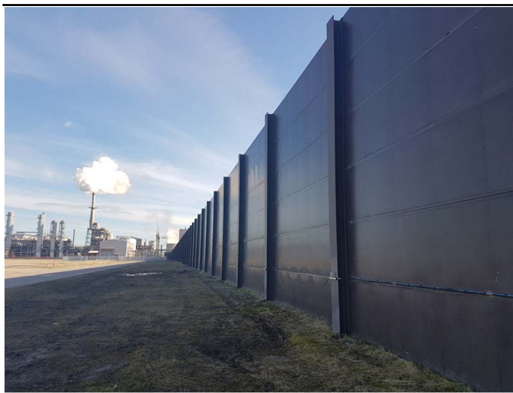
Figure 5.2 Existing Southern Noise Control Wall
